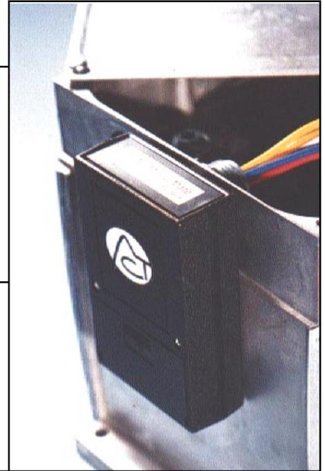
The DRN4 is a resistive output motor actuator interface that accepts several types of DDC system signals. The DRN4 output is 0 to 135 ohms. The input signal types are field selectable by an 8-position DIP switch. Signal input selections include voltage, current, pulse and floating point. Voltage input ranges are 0-5, 1-5, 0-10, or 2-10. Current ranges are 0-20 or 4-20 milliamps. Version 1 pulse input ranges are .59-2.93s, .02-5s, and .1-25.5s. Version 2 pulse input range is .023-
